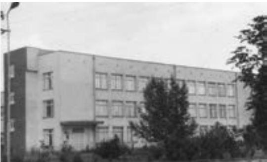
The silkworm egg production facility in Vratsa's building, 1970s (Source / SCS Vratsa archive)
