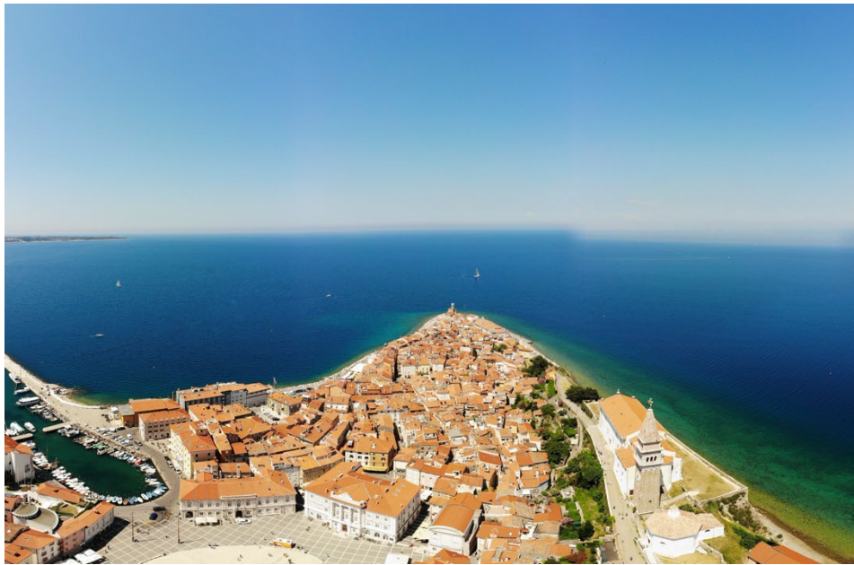
Figure 1: Piran's old town is mostly situated on a low-lying peninsula, making it vulnerable to sea-level rise and storm surges. The northern hilly areas in the picture on the right are prone to flooding during intense rainfall due to impermeable surfaces. Its scenic setting has led to increased tourism and a decline in the local population. These combined factors reduce Piran's resilience to climate change impacts.
