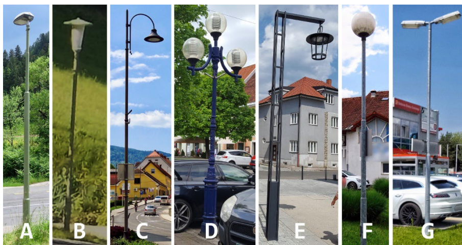
Figure 2: Photographs of different streetlights
