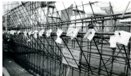
Figure 7. The Soviet documents on rebar. Photo: Rolandas Ginaitis.
