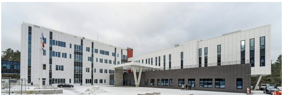
Figure 1. Joint Laboratory Facility for the Faculties of Mechanics, Electronics, and Transport Engineering
