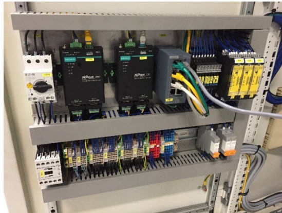
Figure 7: New components mounted on the electrical cabinet door.
