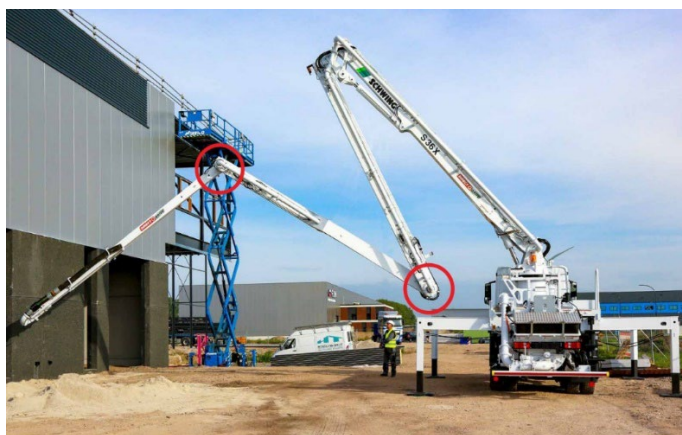
Figure 1: Concrete Pump Boom with two hydraulic motors.
