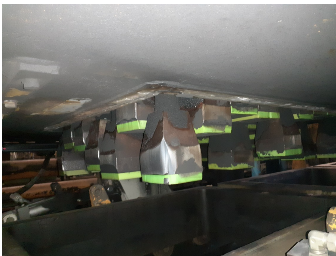
Figure 2: Presence of foundry sand on the press.
